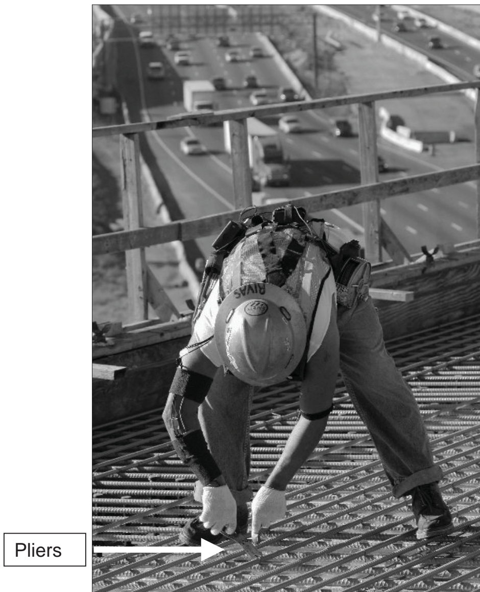
Figure 3 Rebar tying using pliers and tie-wire
